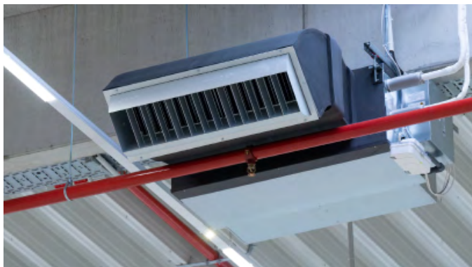
Air outlet with jet nozzles
